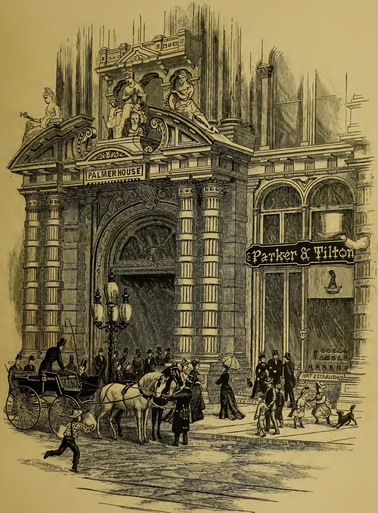
GRAND ENTRANCE PALMER HOUSE, STATE STREET.
